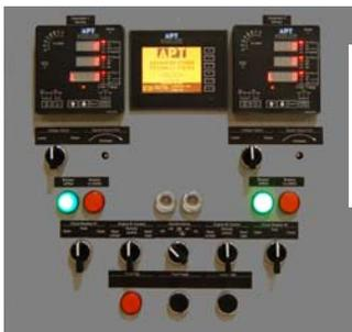
PLC based Control Panels. Generator Paralleling, Load Transfer and Main-Tie-Main Control Panels. Custom Relay Panels.
