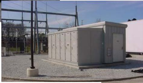
Outdoor walk-in Medium and Low Voltage Switchgear with insulated aisle.
